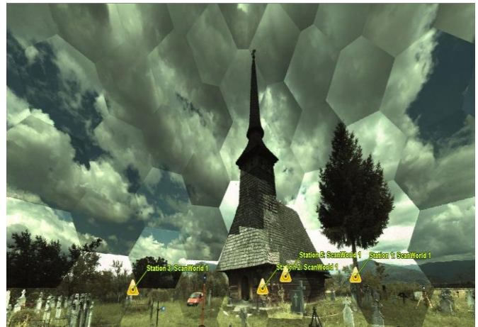
Fig. 6 Stâncești Church – Site map (targets and control points) Full dome image in True View Mode
